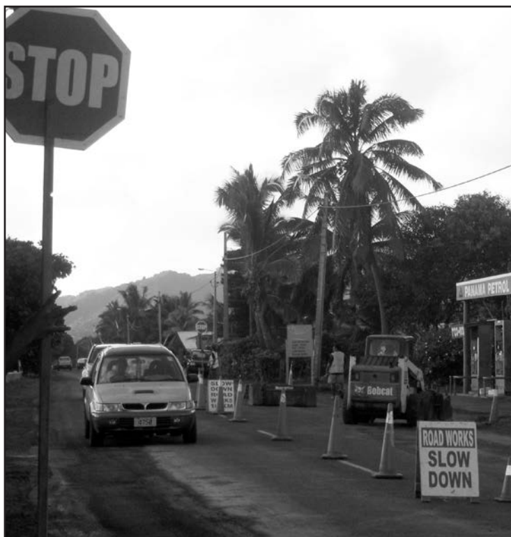
Road Remediation in Panama
