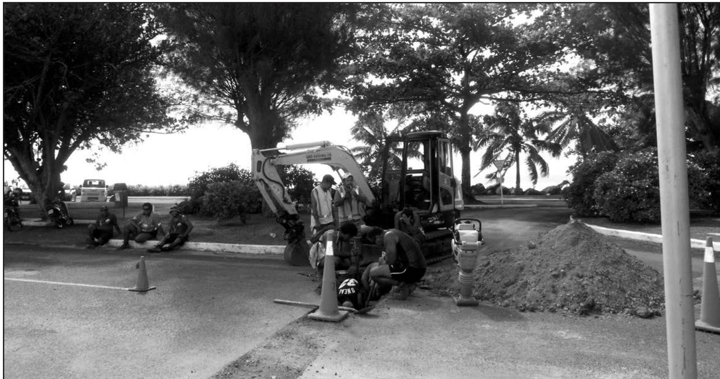
Trenching at Maire Nui rd and the Cooks Corner intersection on Tuesday.
